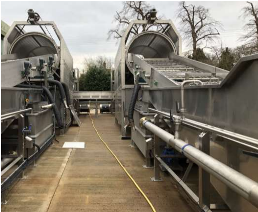
Wash System at Camstar 1
